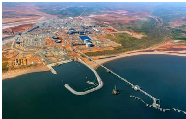
Photo: Steady progress continues at the Wheatstone Project.
