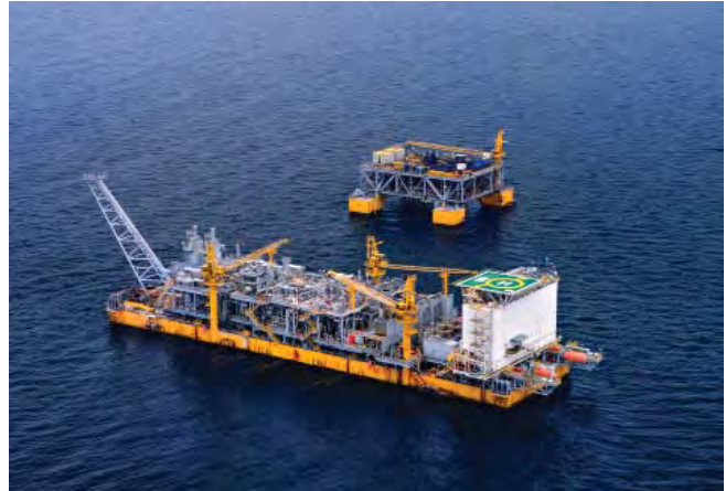
Photo: Production commenced in August 2016 from the Bangka Field, the first stage of the Indonesia Deepwater Development, in East Kalimantan, Indonesia.
