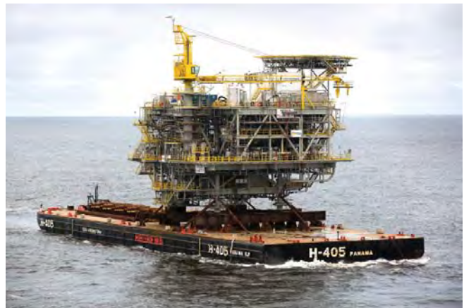
Photo: One of the platform topsides modules is transported to the Mafumeira Sul Field, offshore Angola, prior to installation.
