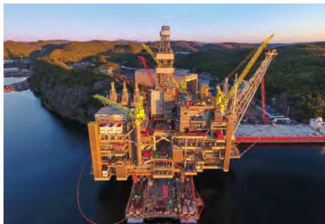
Photo: Topsides for the Hebron platform at Bull Arm, Newfoundland.
