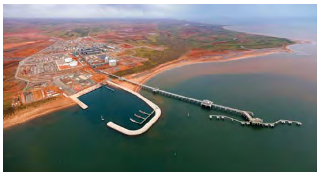
Photo: Construction and commissioning of LNG plant facilities is progressing at the Wheatstone Project in preparation for Train 1 start-up in mid-2017.
