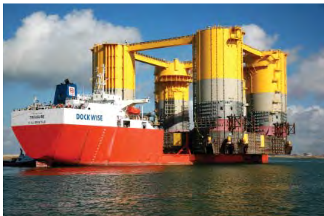
Photo: The hull of the tension leg platform for the Stampede Project arrives at Ingleside, Texas.
