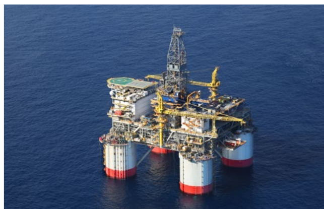
Photo: First oil was achieved from Big Foot in November 2018.
