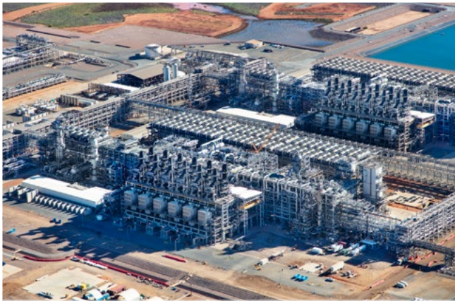
Photo: Start-up of Wheatstone's second train was achieved in June 2018.
