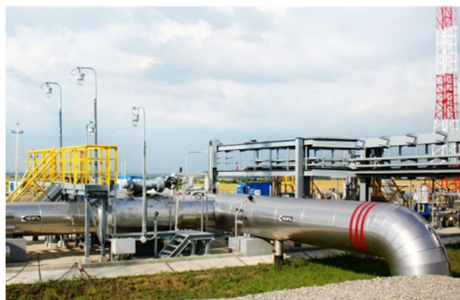
Photo: The CPC pipeline provides a key export route for crude oil production from both TCO and Karachaganak.
